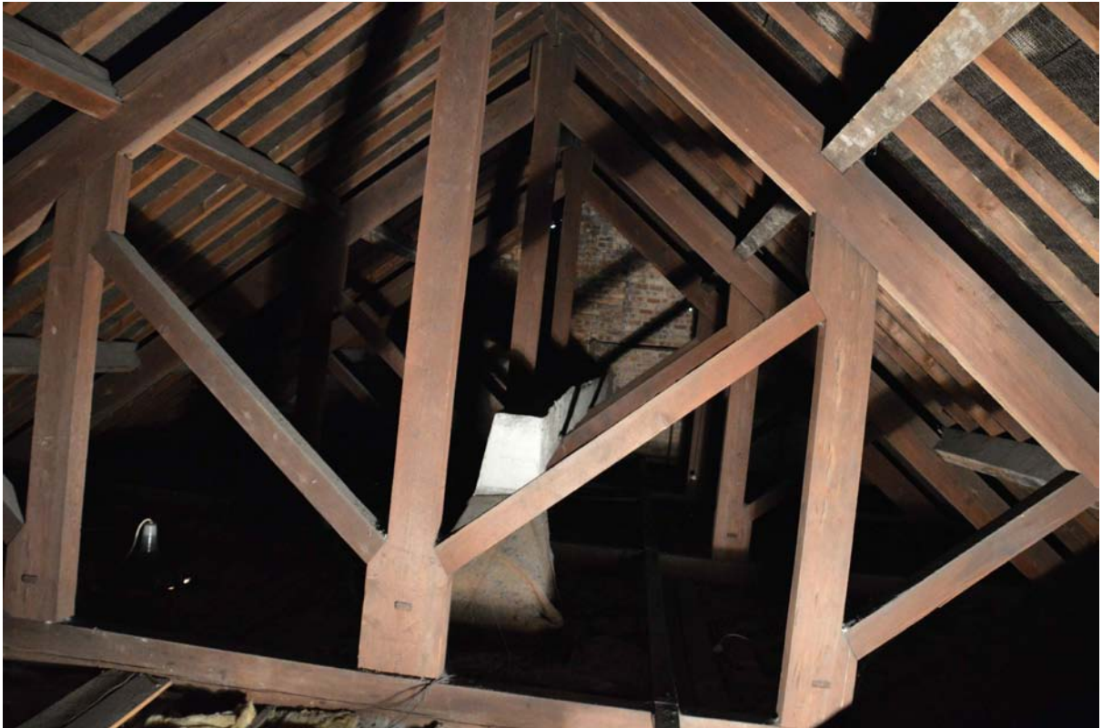
PLATE 65 Timber roof trusses above main body of chapel. Looking east
